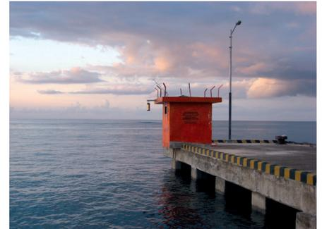
integrated concept was developed, which comprises three different tide gauge sensors and a GPS receiver for vertical control at each site. On-site, the data is quality checked and a detection algorithm for rapid changes in sea level monitors the station independently. All data are transmitted by using GTS/Meteosat and INMARSAT/BGAN. Solar arrays deployed on-site and different communication lines ensure an autonomous operation with minimal maintenance requirements.
